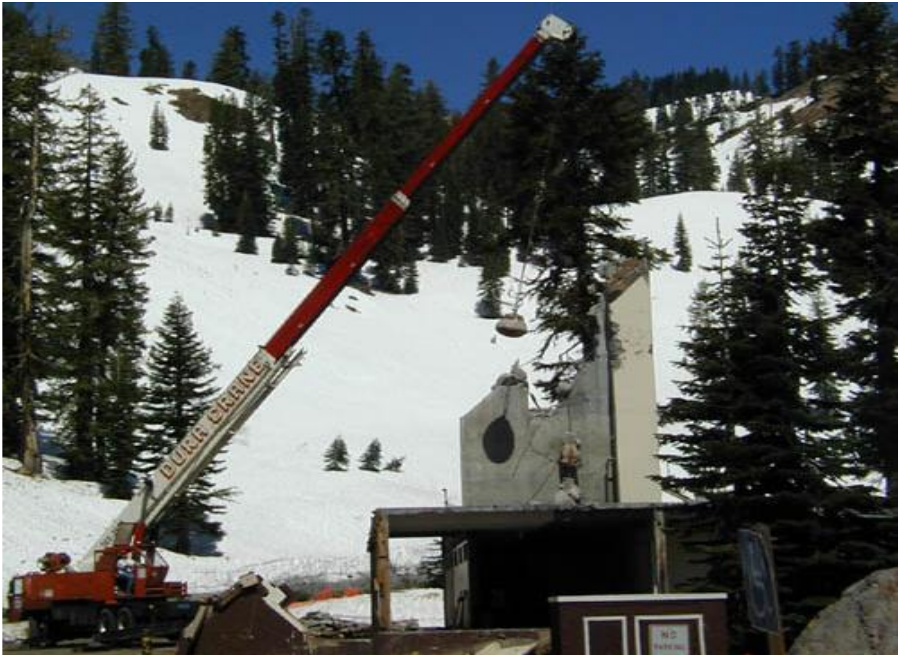
Crane and Wrecking Ball
